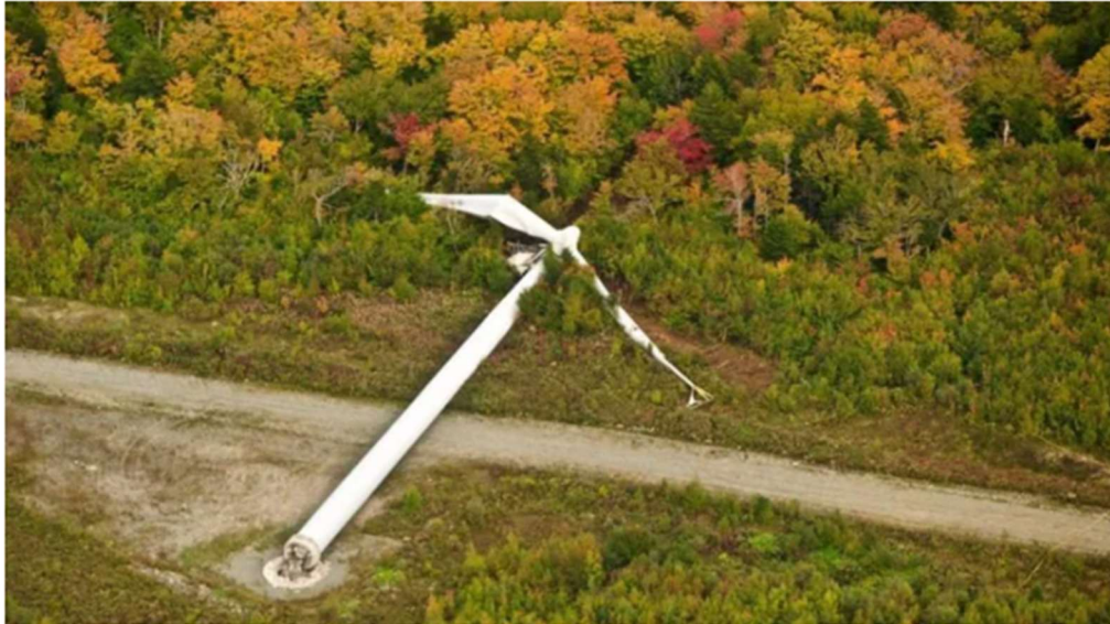
A wind turbine at the Kent Hills wind farm was found collapsed across an access road in September. TransAlta Renewables now says it has found cracks in the foundations of other turbine towers at the site. (Submitted by Steve Shannahan)
